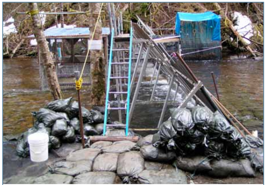
Bipod and picket weir, showing downstream trap to left and upstream trap to right of weir structure at Sitkoh Creek, Chichagof Island.
