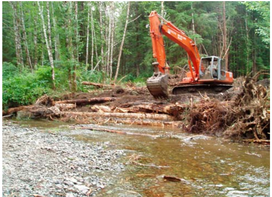
Fubar Phase II Restoration—2007 construction of log jam at meander bend.
