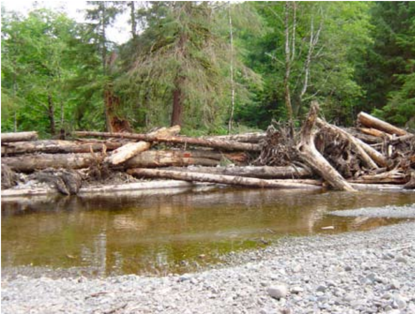
Fubar Phase I Restoration—Large log jam constructed in 2006 (USFS photo).
